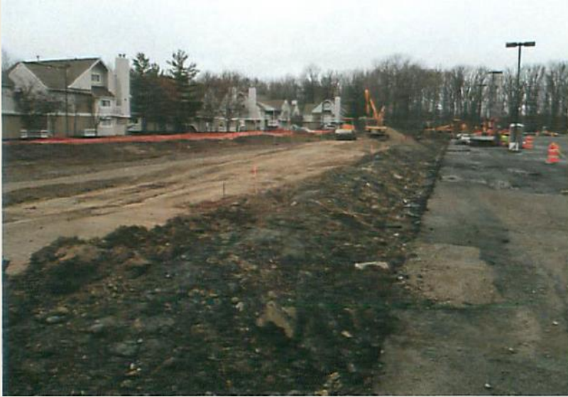
Clemens Road Relocation
