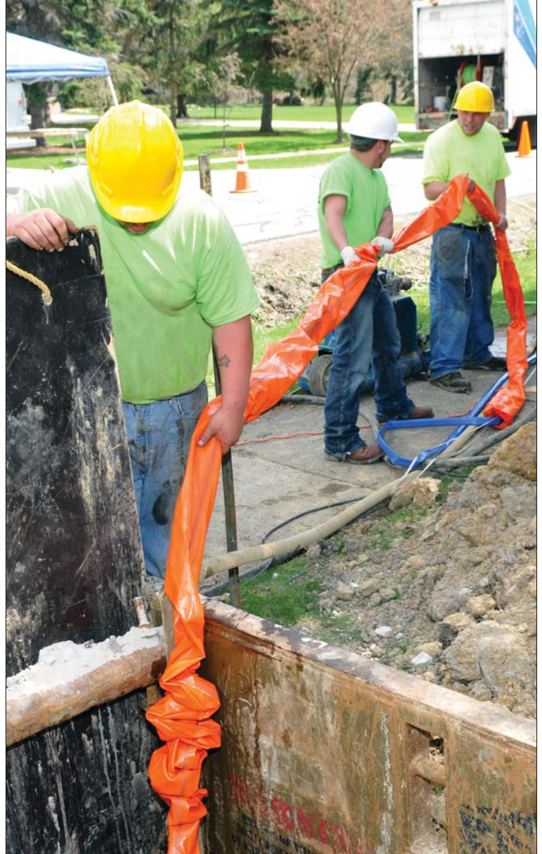
Crew members Neil Sobodinski, Joshua Muron and Bobby Vernatter help extract the calibration bladder assembly, which includes a recycle hose and extraction cord.
