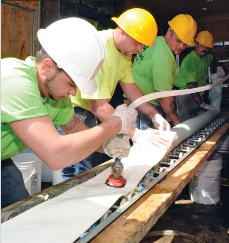
Westlake crew members Joshua Muron, Bobby Vernatter, Neil Sobodinski and Troy Muron work on the wet-out assembly line on a CIPP lining project.
