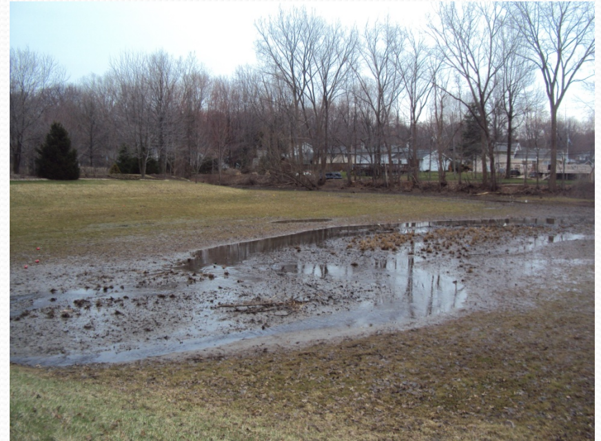
SOUTHBRIDGE RETENTION BASIN
