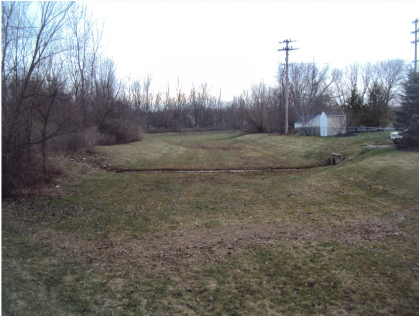
SHERWOOD RETENTION BASIN
