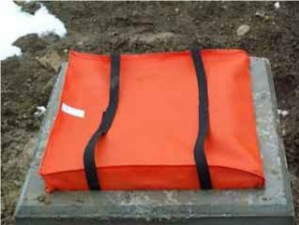
Manufactured filter bag over flat grated inlet
