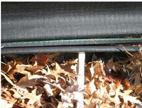
Fabric not tucked into soil
