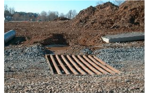
Stabilized construction entrances allow dirt to be removed from tire treads and collected as trucks leave construction sites
